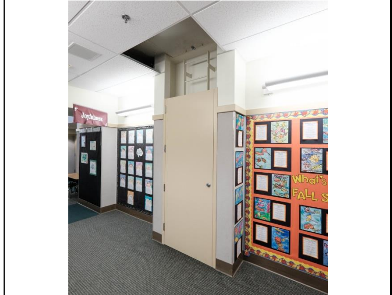
Photo 16 Building Name: Admin/Classroom Building Building Number: 1 Roof access from corridor
