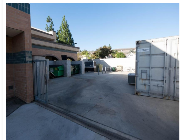
Photo 20 Building Name: Admin/Classroom Building Building Number: 1 Trash enclosure adjacent to Building 1 on east side.
