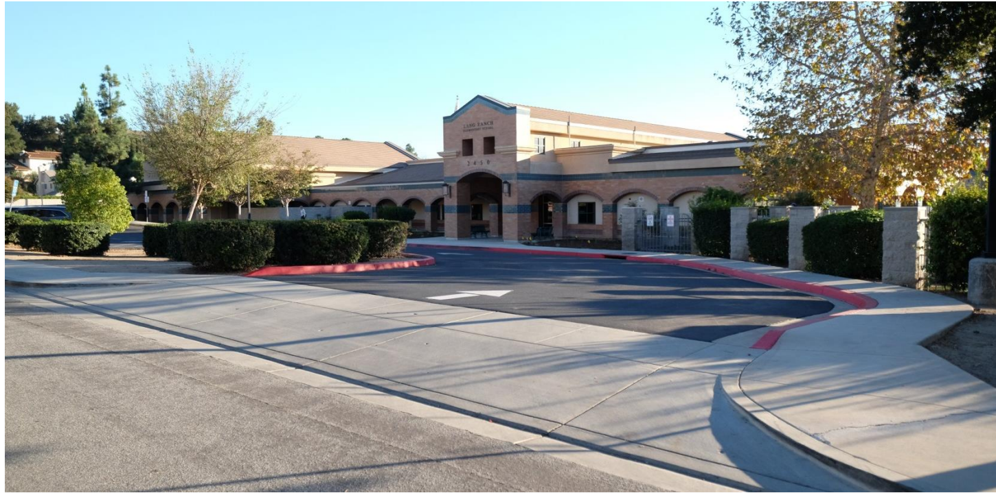
Image 1: Main entry from Whitechapel Street
