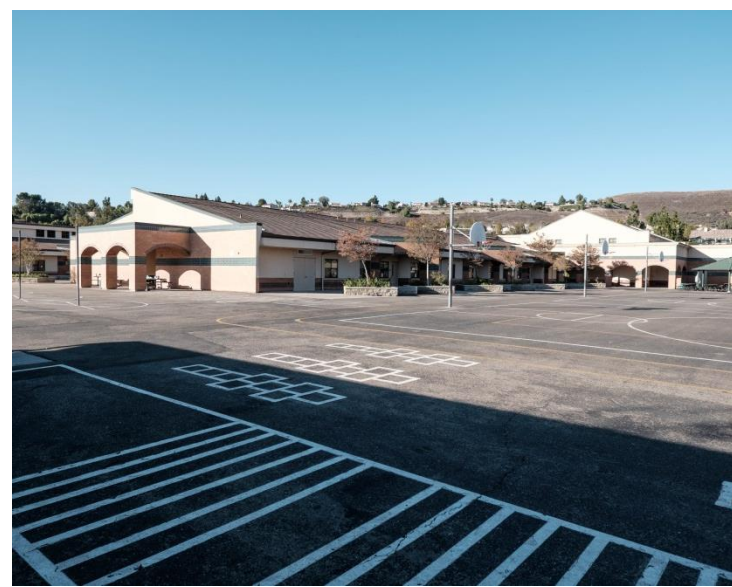
Photo 2 Building Name: Admin/Classroom Building Building Number: 1 View of east wing from basketball courts.
