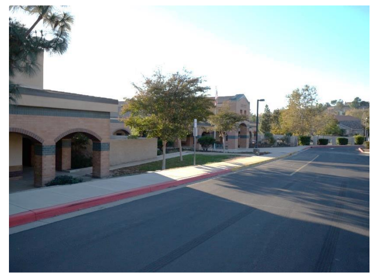
Photo -4 Circulation to main School Building slightly sloping.
