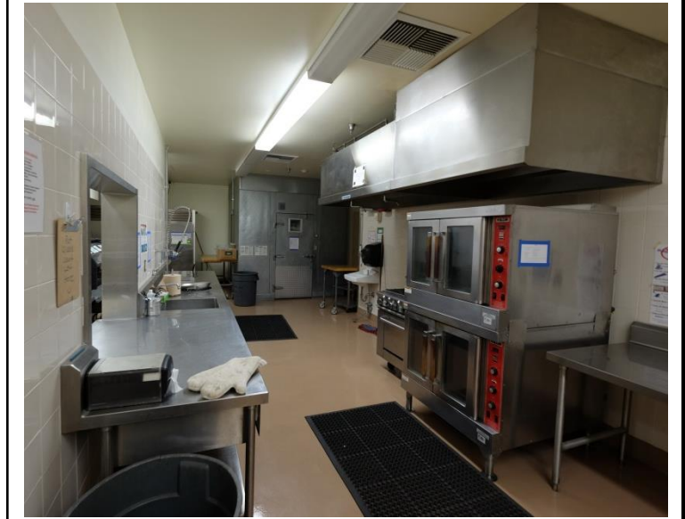
Photo 12 Building Name: Admin/Classroom Building Building Number: 1 Kitchen
