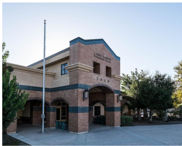
Photo 1 Building Name: Admin/Classroom Building Building Number: 1 Entrance to lobby.
