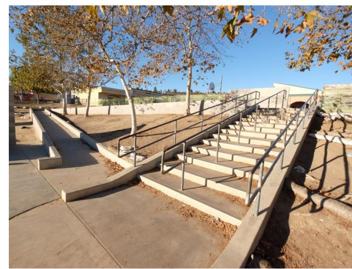
Photo -3 Ramp and stairs down to Building 6 and lower athletic field.
